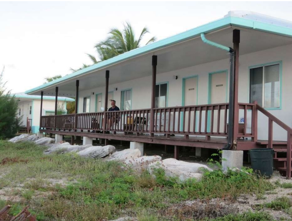
Diver accommodation block.
